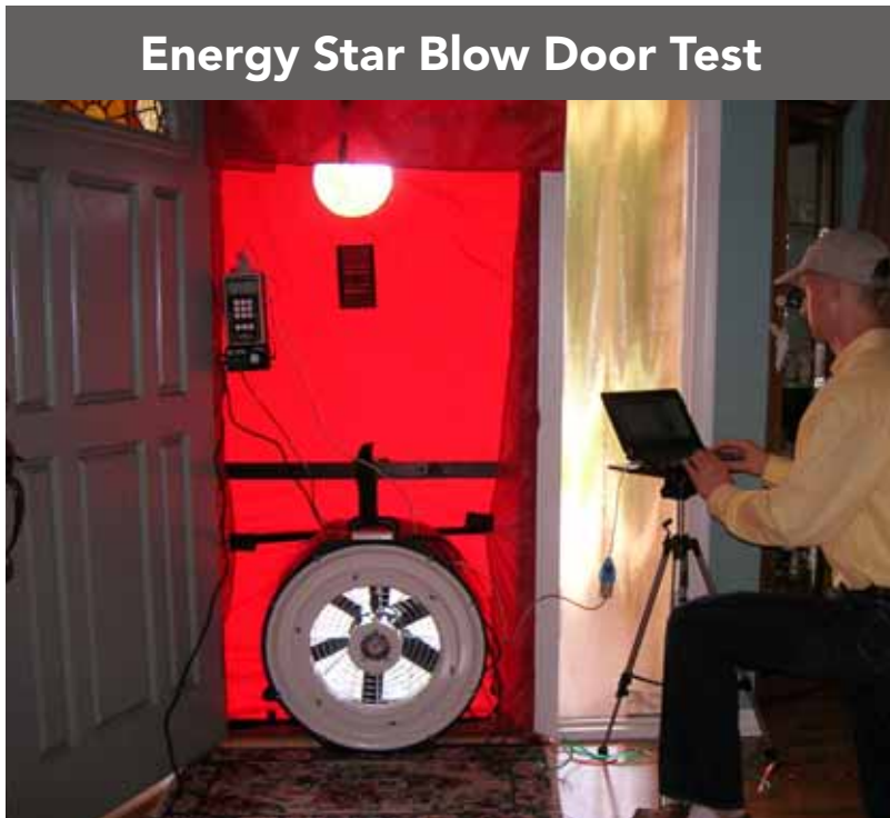
An independent third-party conducts a blow door test to confirm the air tightness of your home. This would be a good time to contact your solicitor and financial institution to ensure everything is in order for your closing day.
