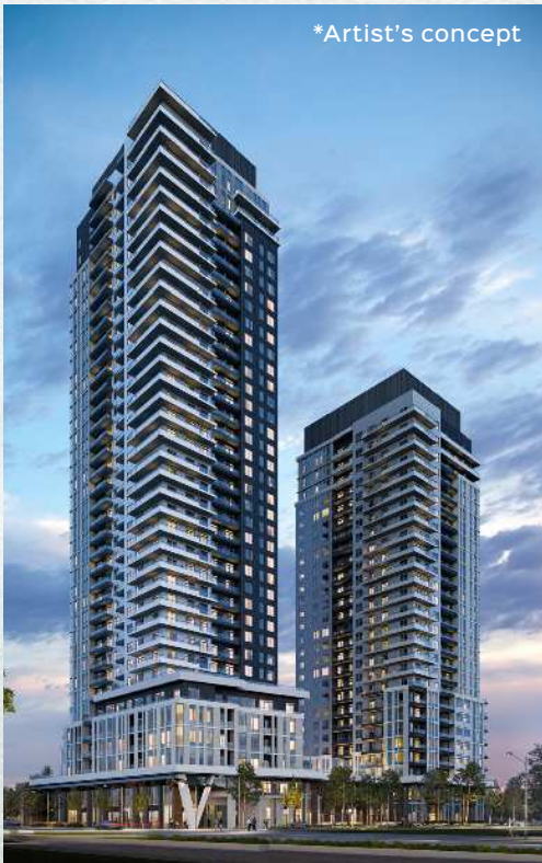
The Vincent VAUGHAN Under Construction
